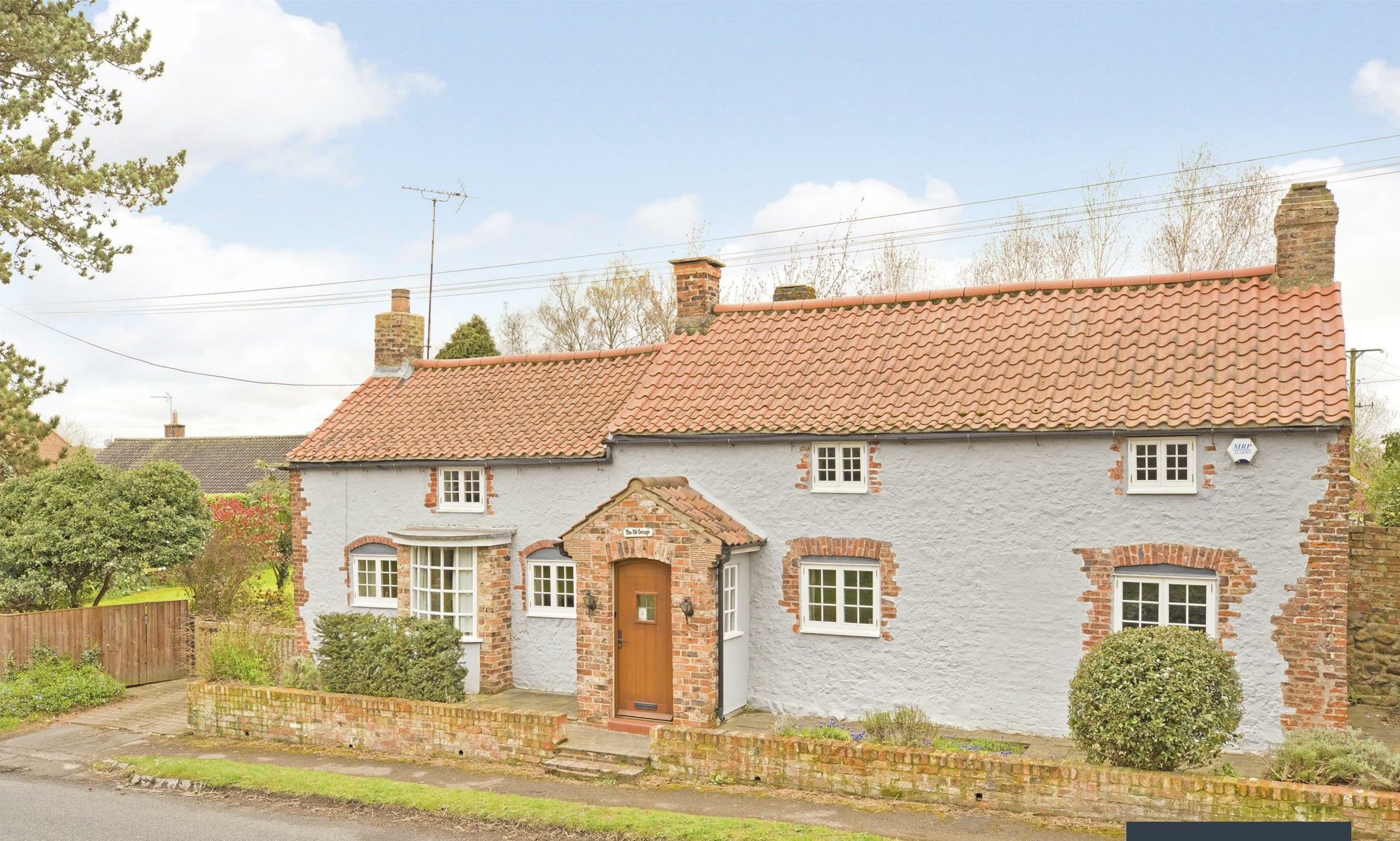
THE OLD COTTAGE Main Street, Little Ouseburn
