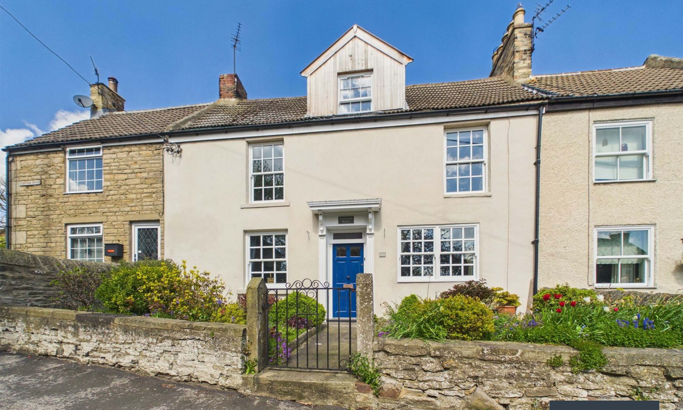
KIRKSTONE HOUSE 22 STATION ROAD Witton Le Wear
